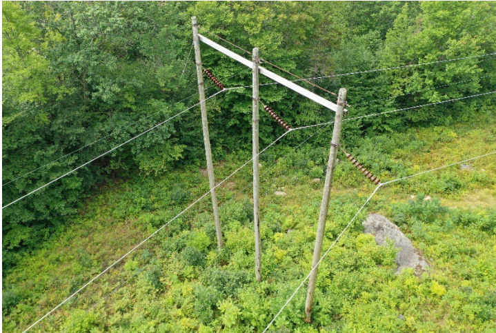
Examples of existing structures to be removed
