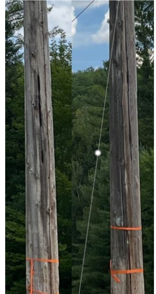
Cracked Pole
