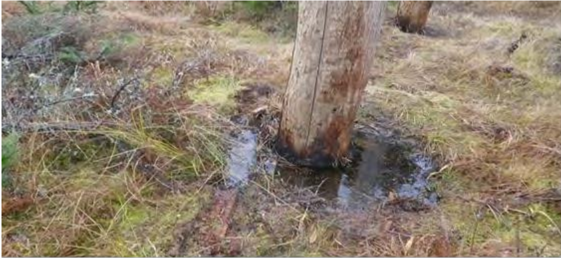
#224 cross arm not removed to reduce wetland impacts
