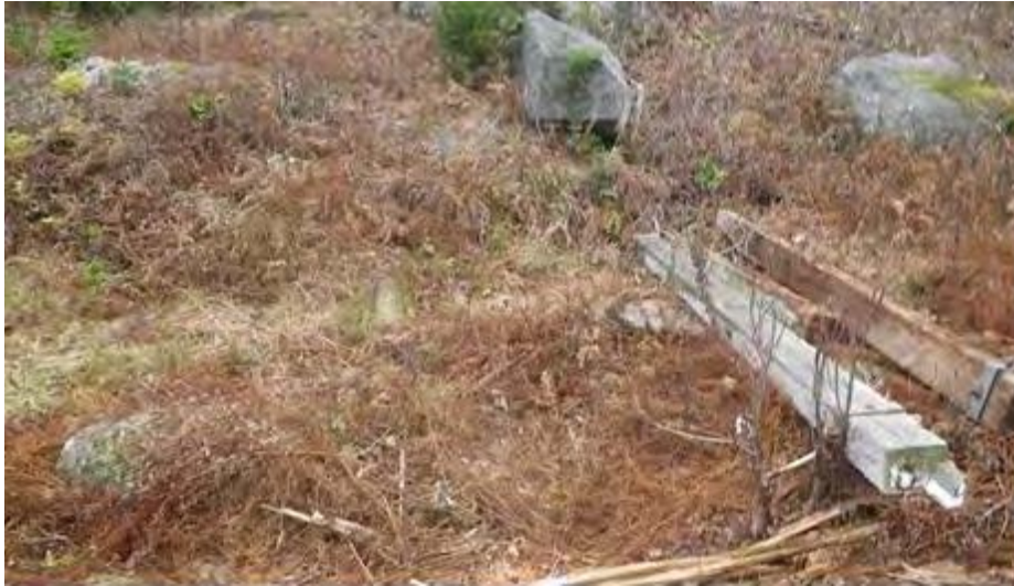
STR 243 cross arms awaiting removal – 11/2/15
