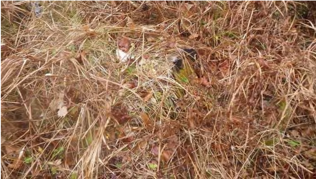
#273 – pole piece buried in wetland, not removed
