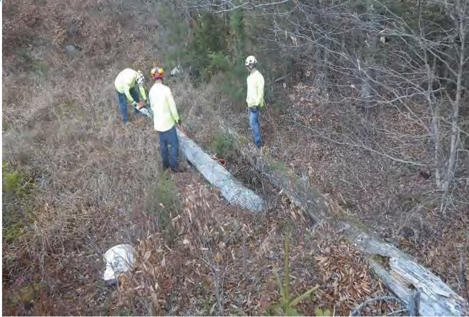
Poles at #214 prior to removal
