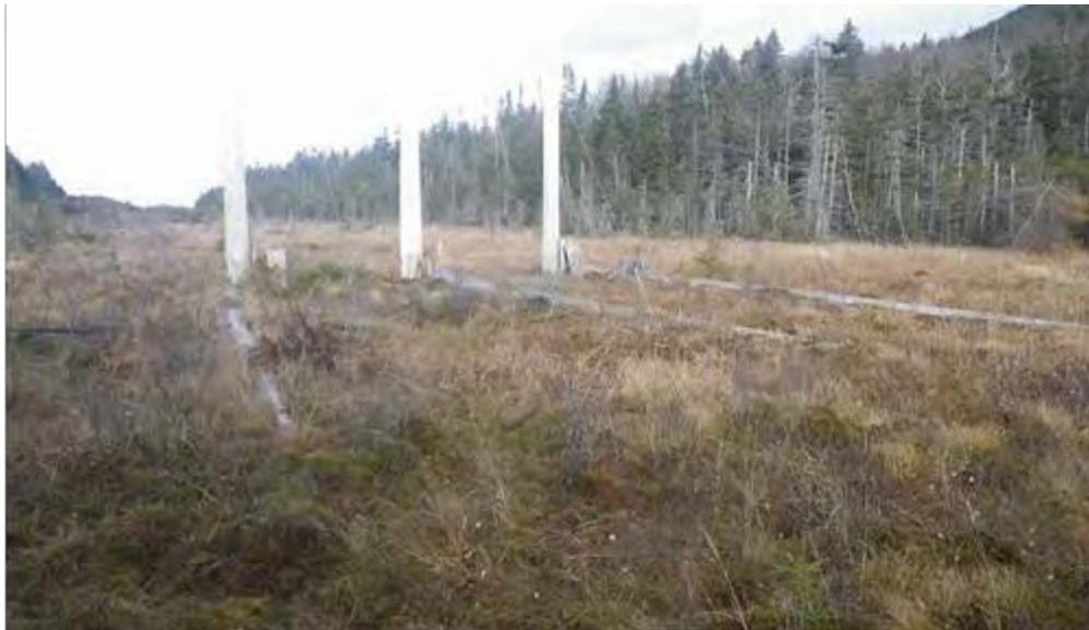
Poles left in wetland near structure 264 to avoid wetland impacts – 11/3
