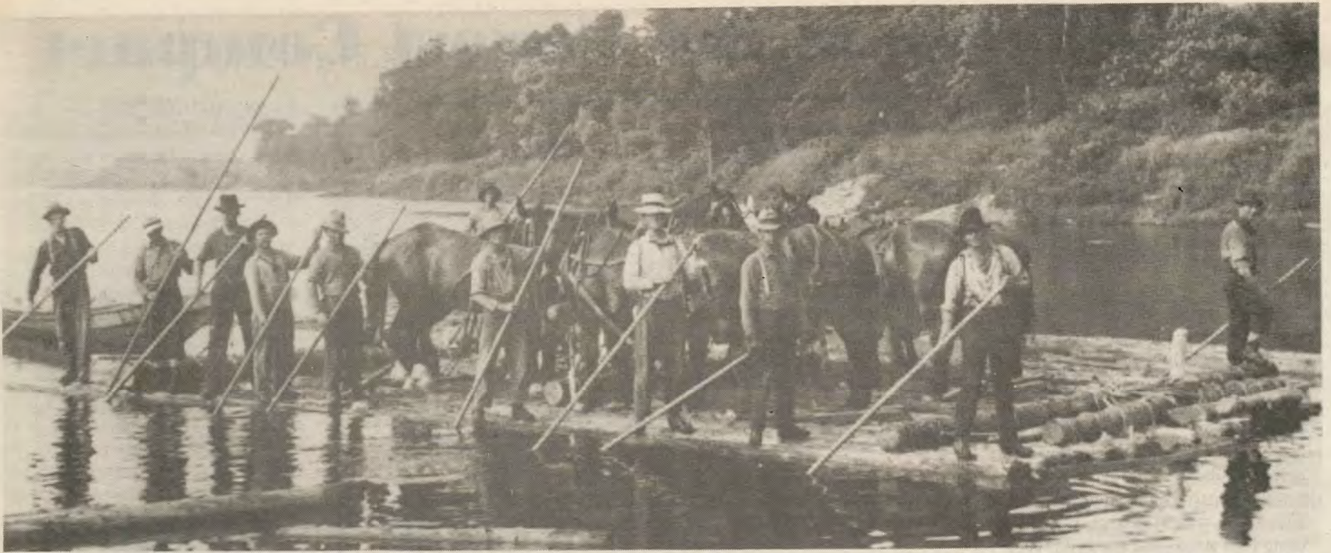
The famous 'horse-raft' that was used to drag stranded logs off the ledges and banks in the Connecticut River near North Stratford and the Nulhegan River. From 200th Anniversary of Stratford, NH.
