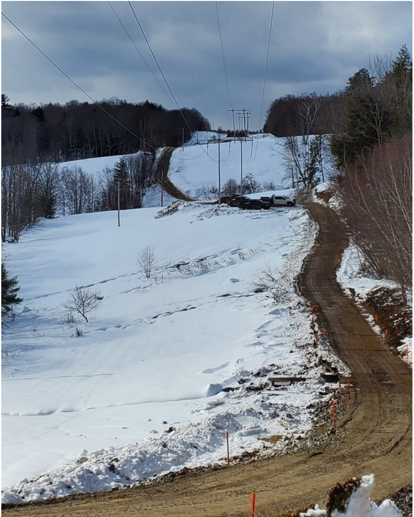
Road Construction on the E-115 line:
