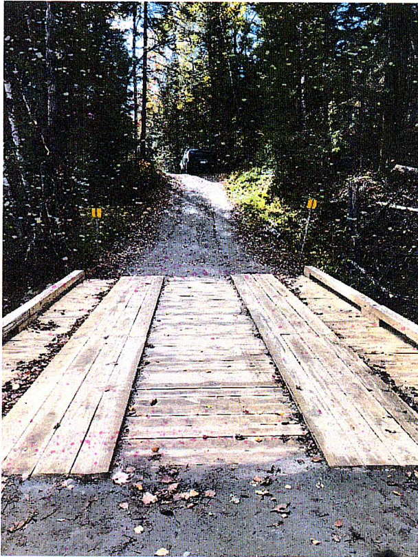
Figure 1- Newly built bridge
