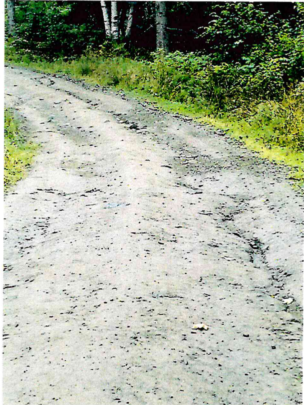
Figure 4 and 5- Shows some of the wear on the trail heading toward Colebrook.
