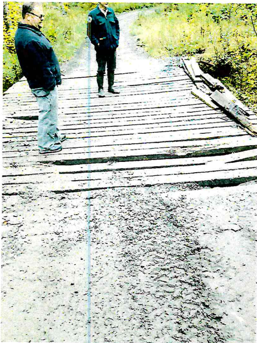
Figure 10- Depicts the repaired approach to the bridge, however, still shows the decking that needs replacing.
