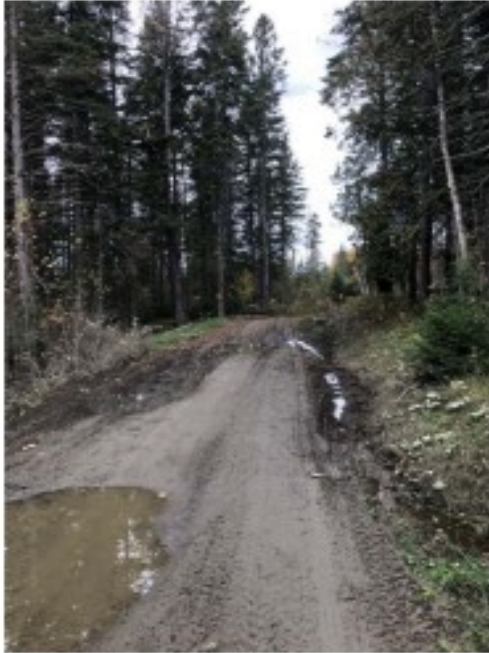
Figure 4- Mud on trail and ATV tracks in ditch and minor sedimentation on trail from water.
