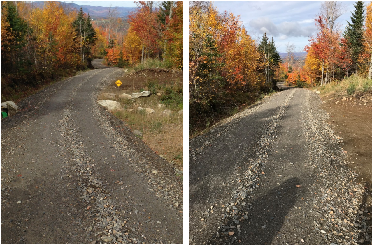
Figure 10 and 11- Depicts the newly graveled section of trail.
