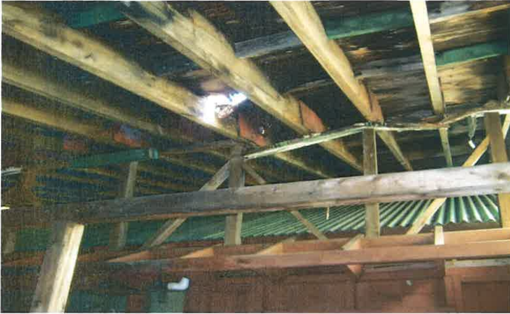
Interior of bathhouse
