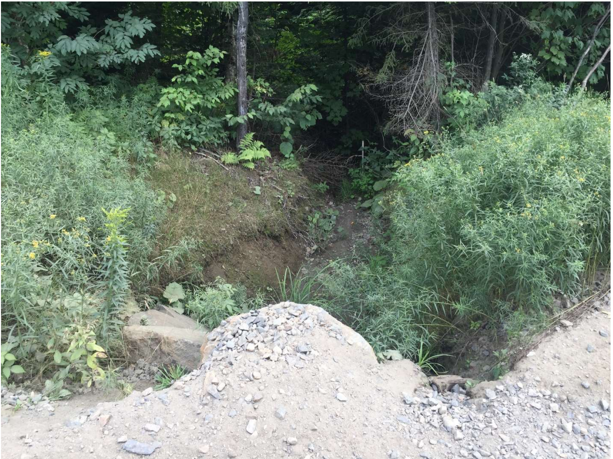
New Gravel covering Erosion
