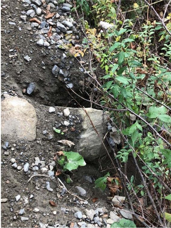
*Figure 6- Depicting the area where the water is eroding around the culvert.*
