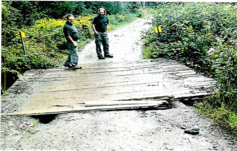
Figure 1, 2 and 3- Shows the broken boards on the bridges and the eroding approaches.
