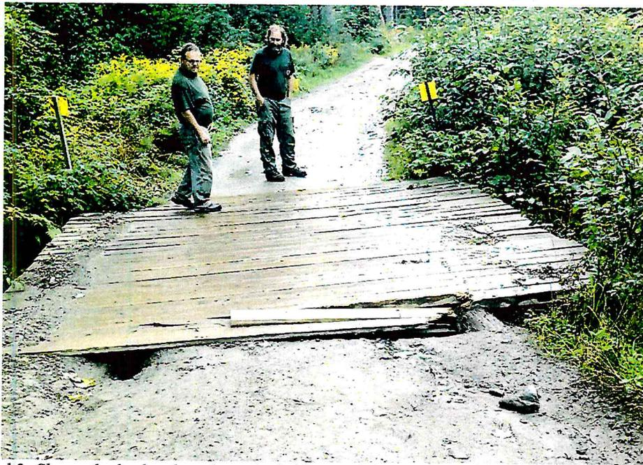
Figure 1, 2 and 3- Shows the broken boards on the bridges and the eroding approaches.
