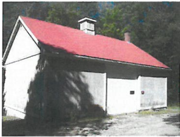
barn on site
