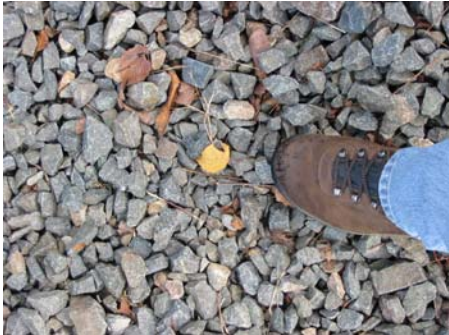
Railroad ballast, Northern Railroad, Boscawen
