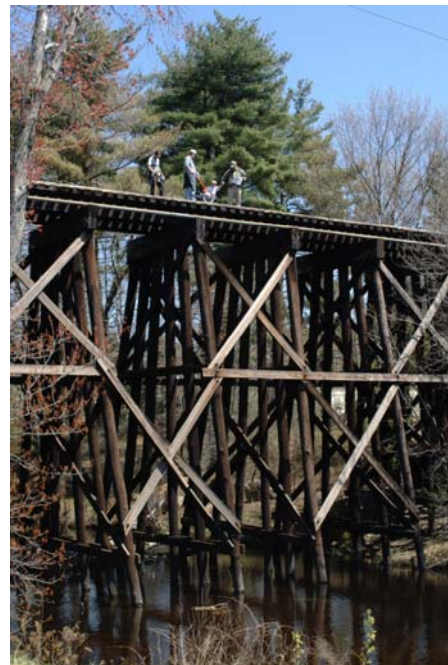
Rail Bridge over Massabesic River, Manchester
