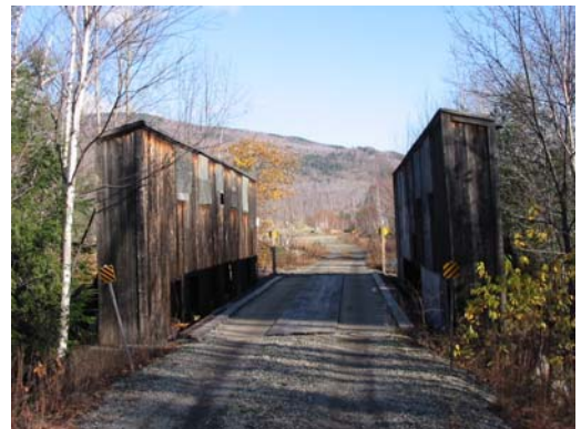
Boxed Pony Truss Bridge on Rail Trail
