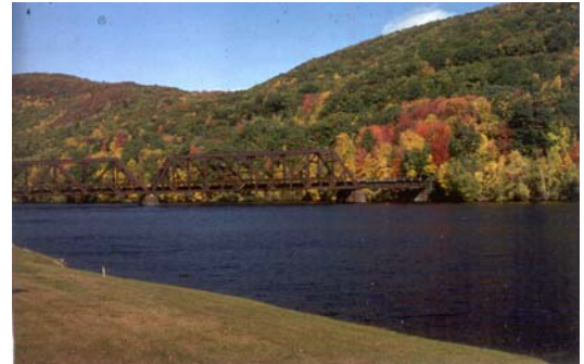
Rail bridge over Connecticut River
