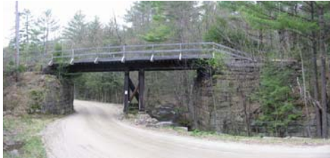
Rail bridge over Roy Ford Road in Danbury
