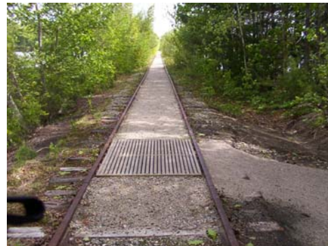
Area between rails filled in for trail use
