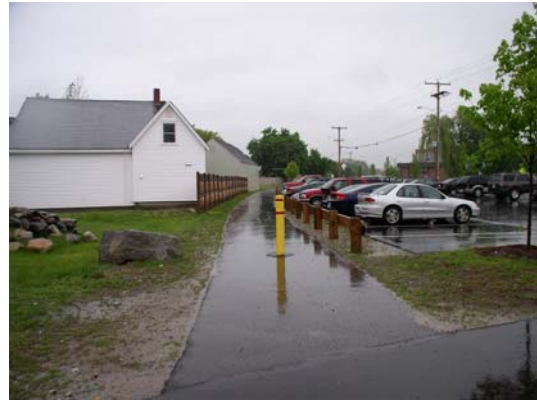
The Farmington Branch (aka Lilac City Greenway) runs through downtown Rochester with some paved segments
