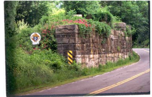
Rail bridge abutment
