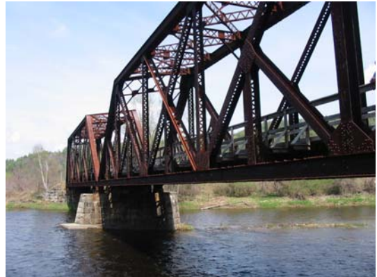
Rail bridge over Ammonoosuc River in Lisbon
