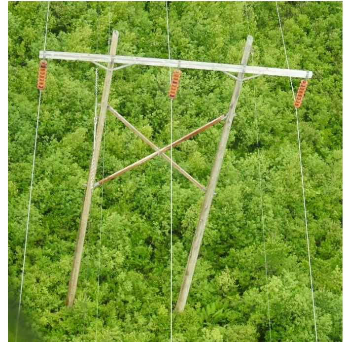
Typical Wood Structures
