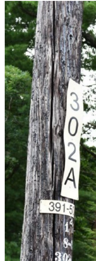
Line 391-508 – Structure 302A
