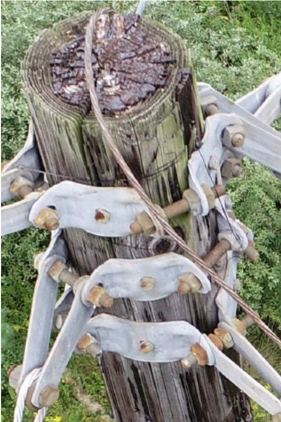
Line 533-508 – Structure 270A
