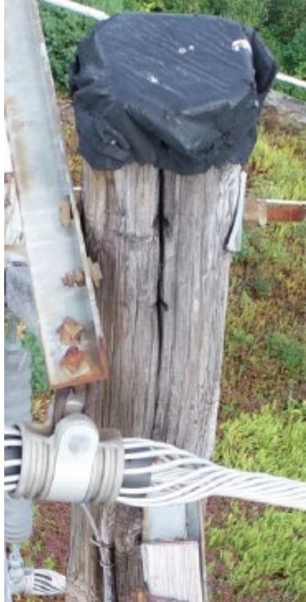
Line 211-508 – Structure 359A
