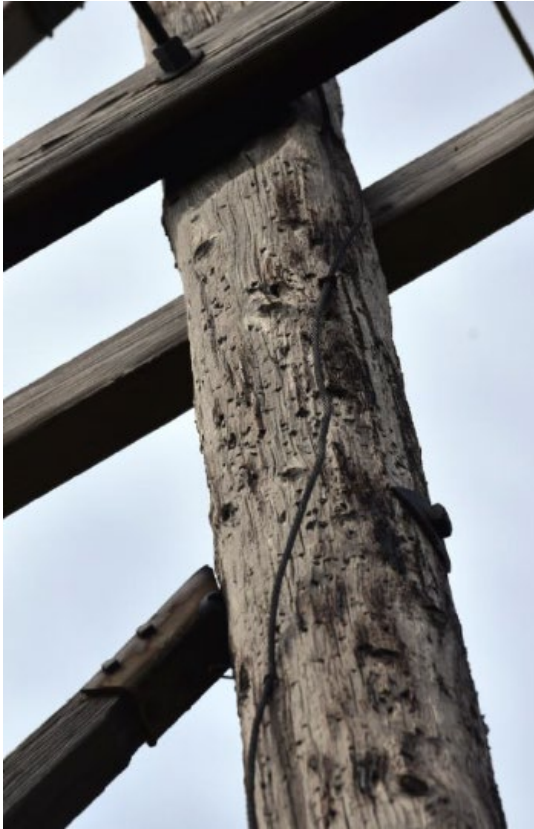
Line 391-508 – Structure 308A
