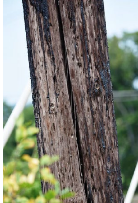
Line 211-508 – Structure 318A
