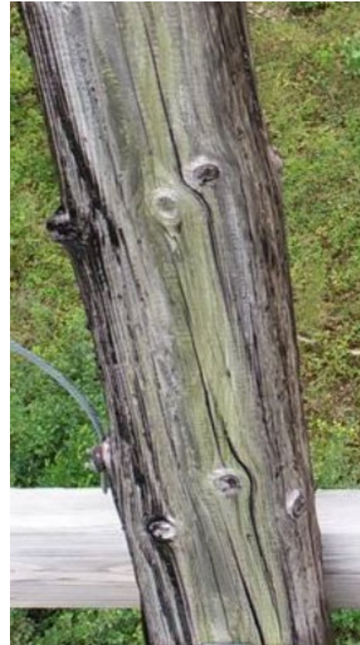
Line 533-508 – Structure 280A
