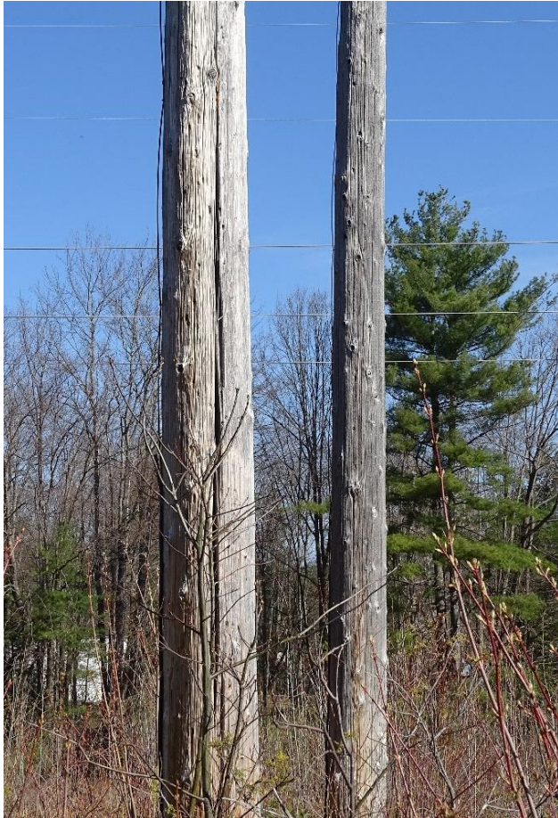
C196 Line – Pole Splitting
