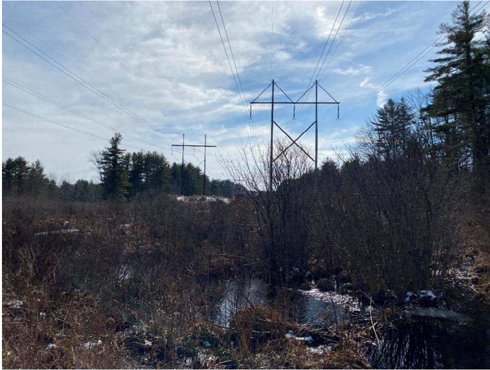
Photograph No. 17: Looking at proposed access and work pad location adjacent to 373 Structure 264.
