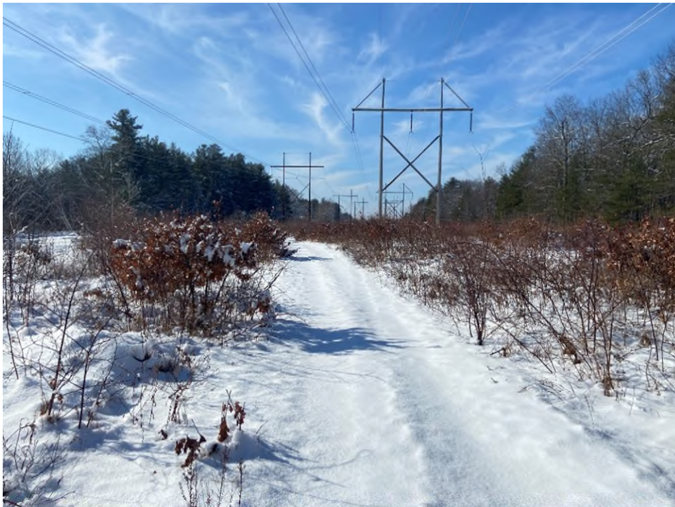
Photograph No. 4: Looking at proposed access and work area for 373 Structure 318.
