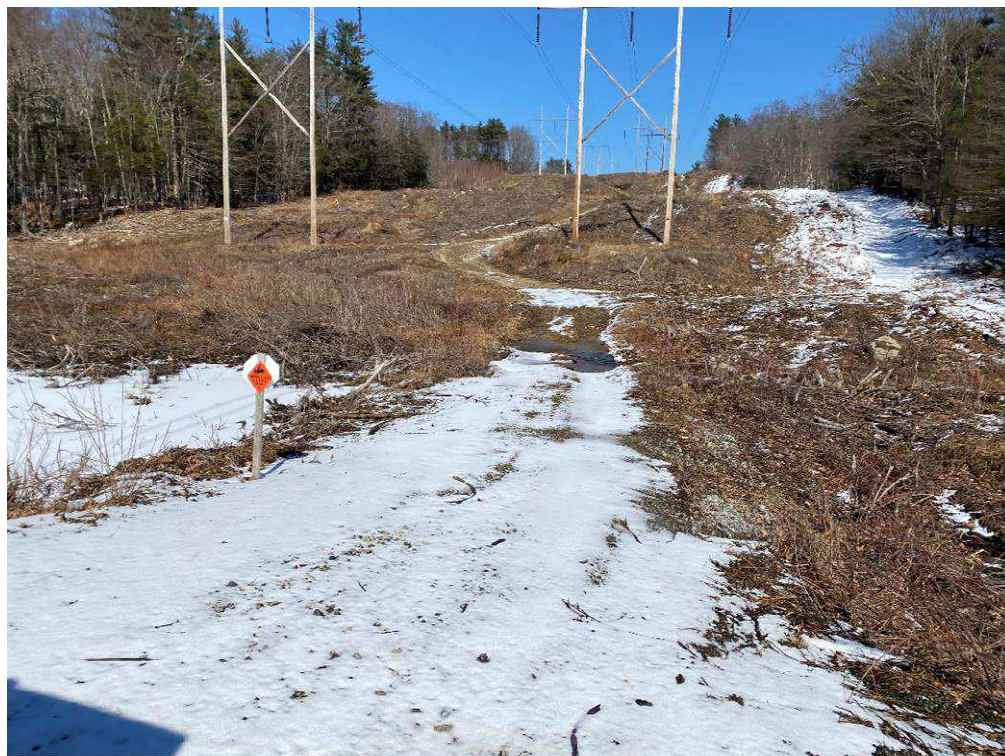
Photograph No. 36: Looking at proposed access to 385 Structure 127.
