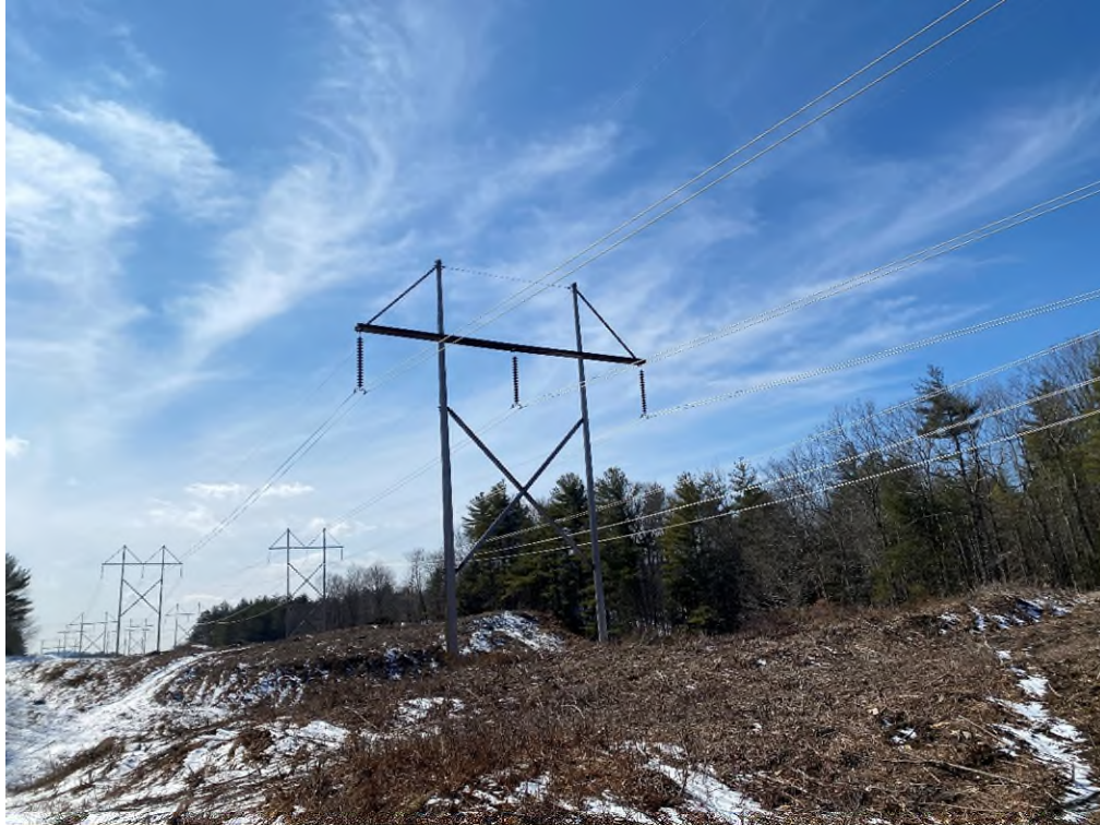
Photograph No. 33: Looking at proposed access to 373 Structure 145.
