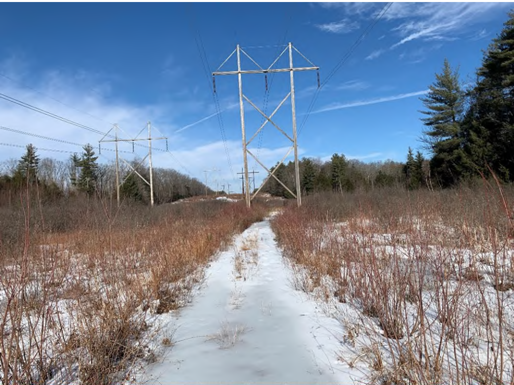
Photograph No. 10: Looking at proposed access and work pad location for 373 Structure 297.
