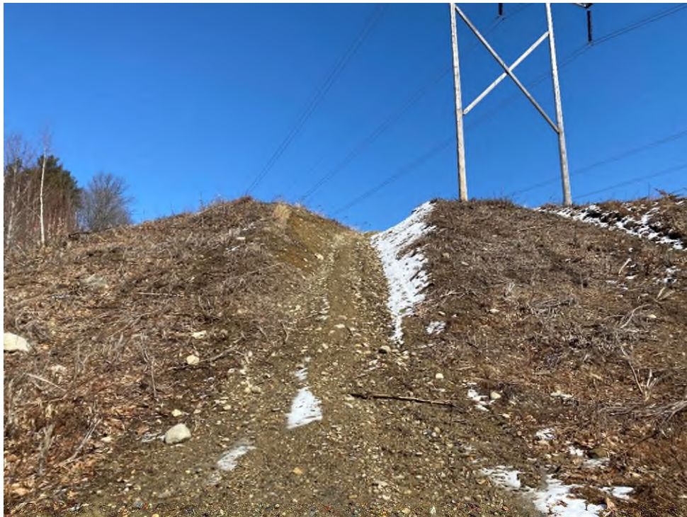
Photograph No. 38: Looking at proposed access for 385 Structure 126.
