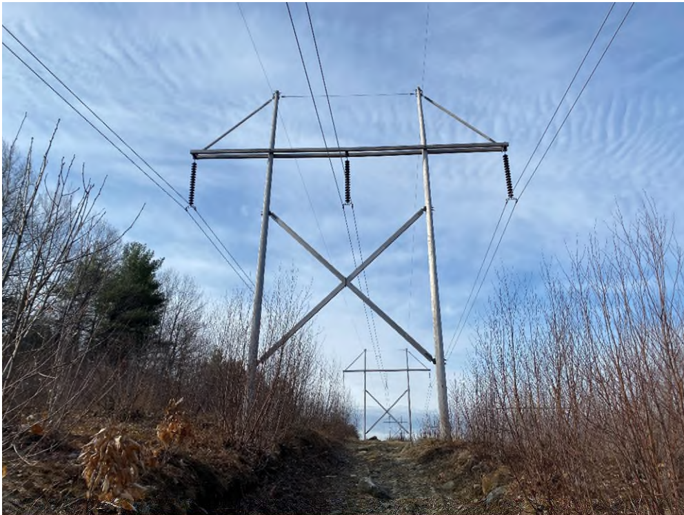
Photograph No. 26: Looking at proposed access and work pad location for 391 Structure 191.
