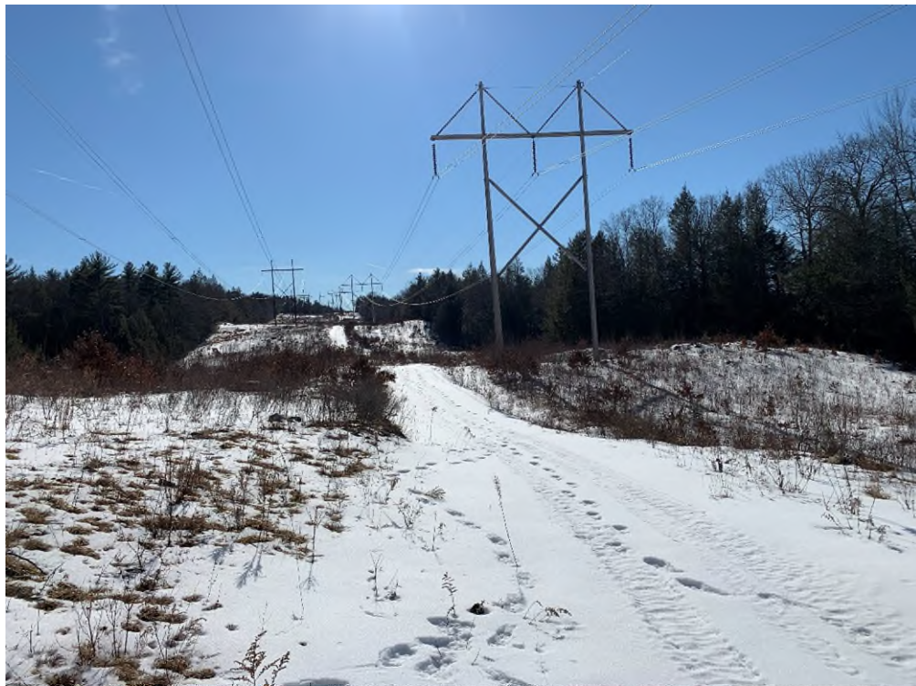
Photograph No. 8: Looking at proposed access and work pad location adjacent to 373 Structure 299.
