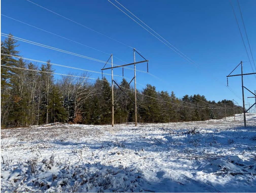
Photograph No. 61: Looking at proposed access and work pad location adjacent to 385 Structure 34.
