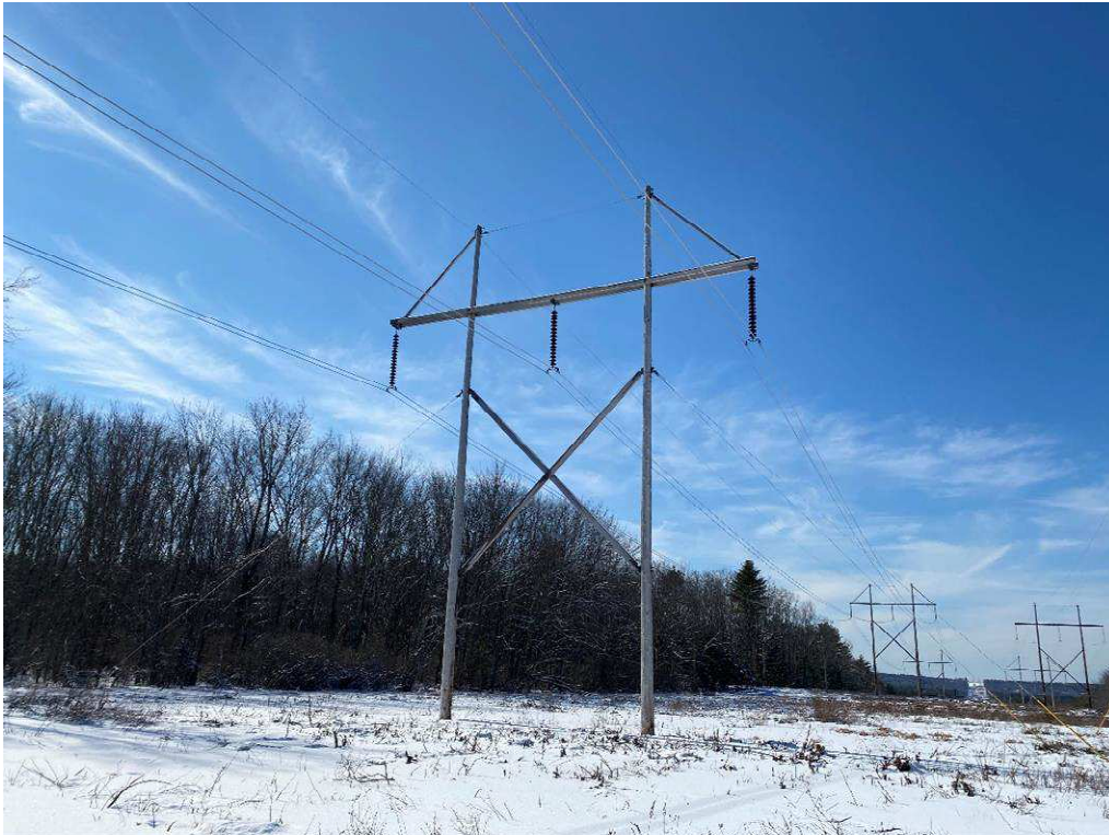
Photograph No. 51: Looking at proposed access and work pad location for 391 Structure 76.
