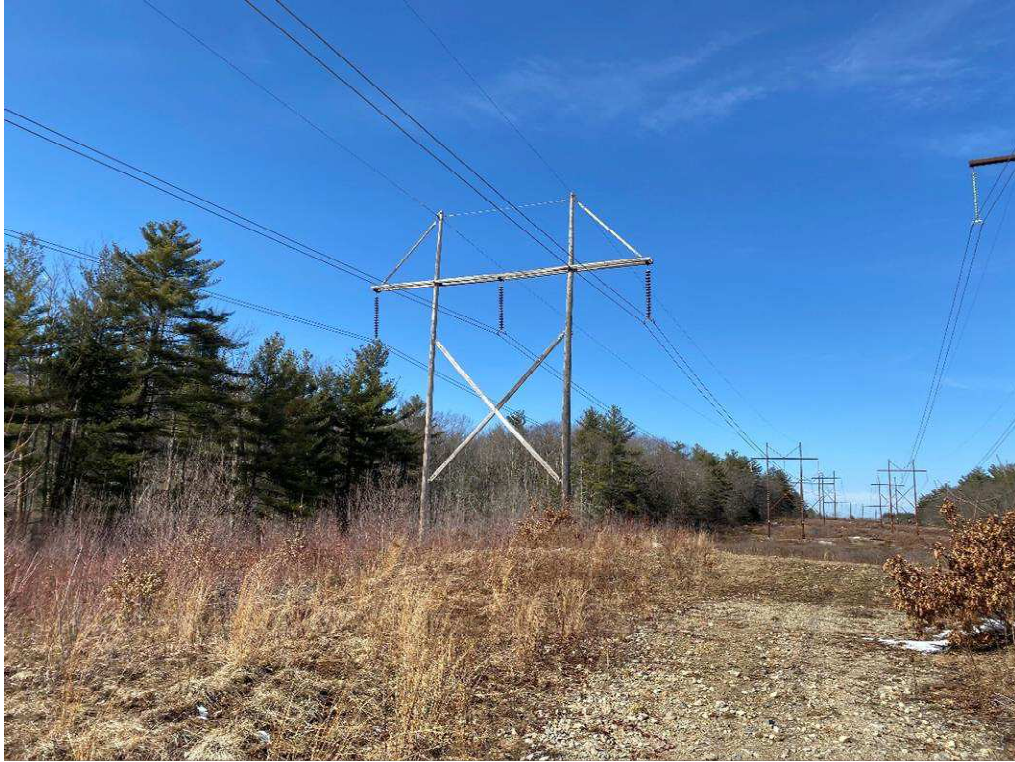
Photograph No. 21: Looking at proposed access and work pad location for 373 Structure 255.
