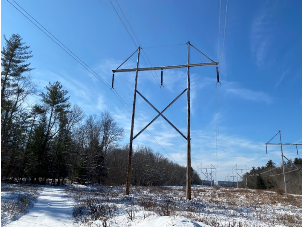
Photograph No. 53: Looking at proposed access and work pad location for 391 Structure 75.
