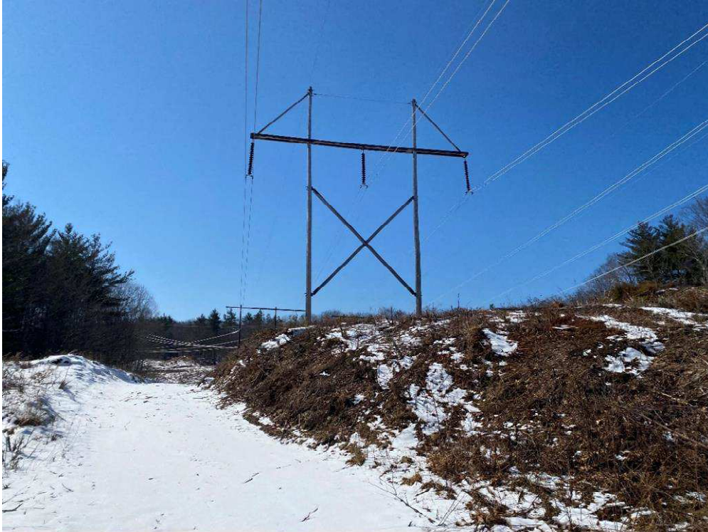
Photograph No. 41: Looking at proposed access to 391 Structure 121.
