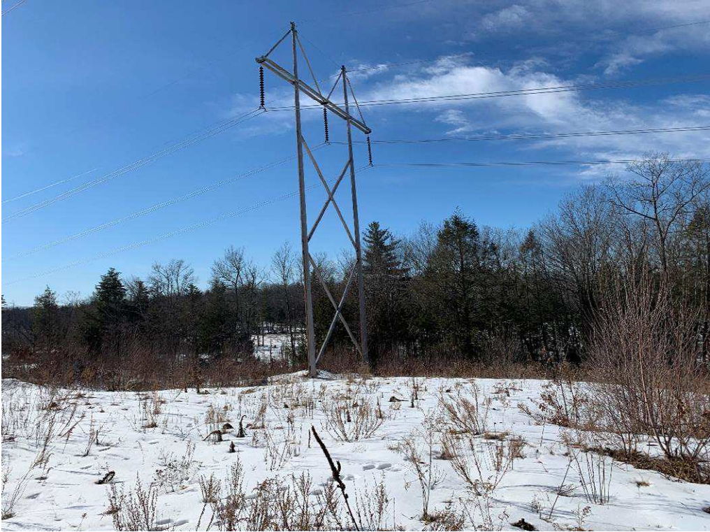
Photograph No. 9: Looking at proposed access and work pad location adjacent to 373 Structure 298.
