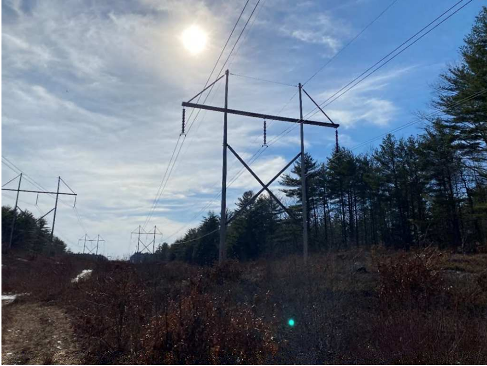
Photograph No. 19: Looking at proposed work pad location for 373 Structure 262.
