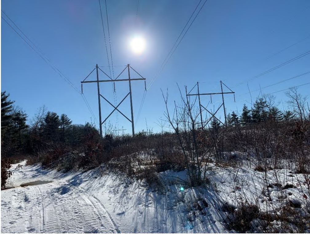
Photograph No. 13: Looking at proposed access for 391 Structure 132 and 373 Structure 276.
