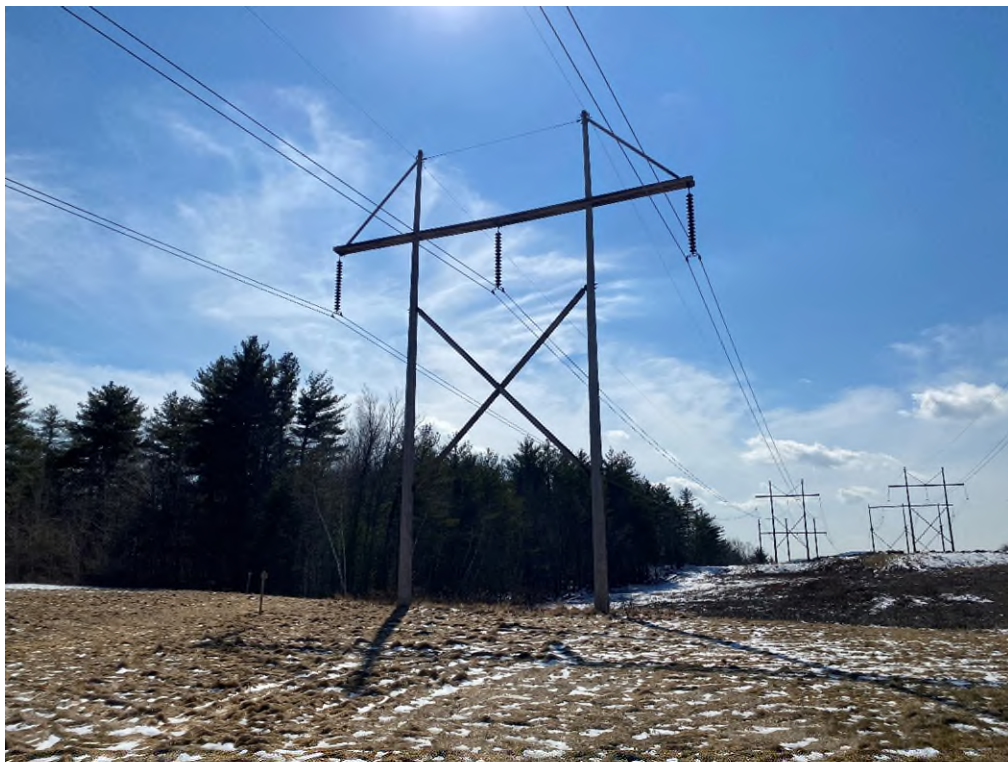
Photograph No. 30: Looking at proposed access and work pad location for 373 Structure 147.
