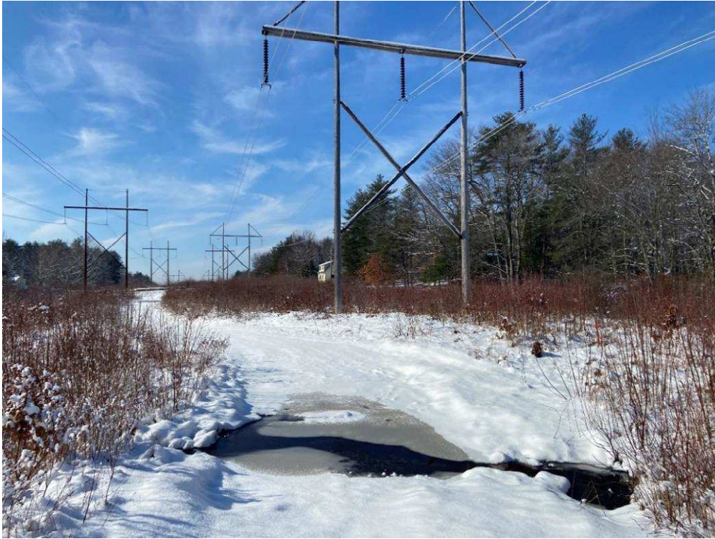
Photograph No. 3: Looking at proposed access and work pad location for 373 Structure 319.
