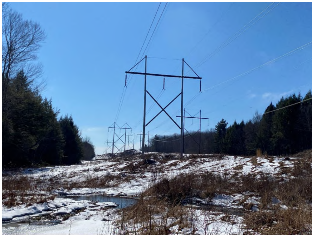
Photograph No. 34: Looking at proposed access to 391 Structure 133.
