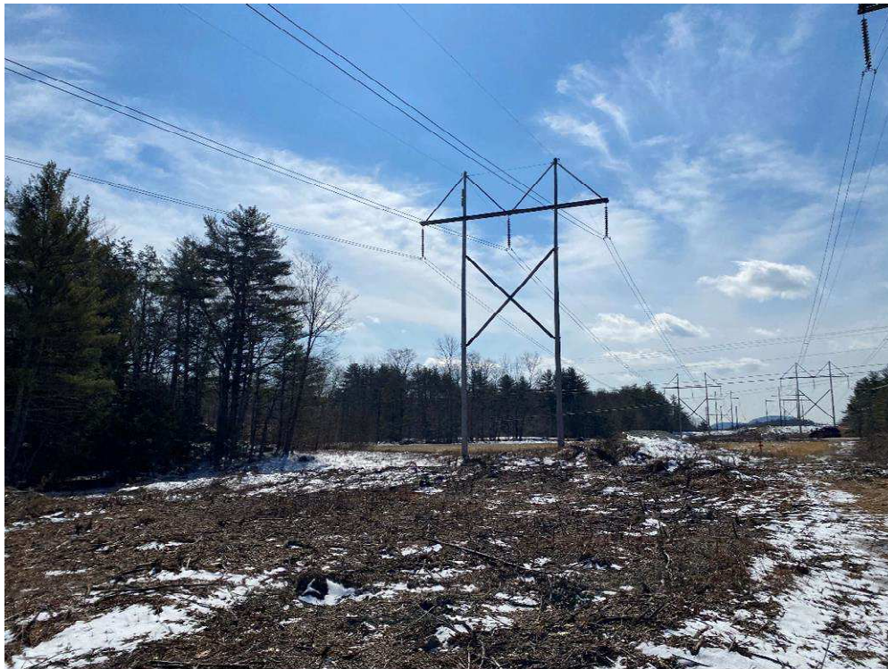
Photograph No. 32: Looking at proposed access to 373 Structure 146.
