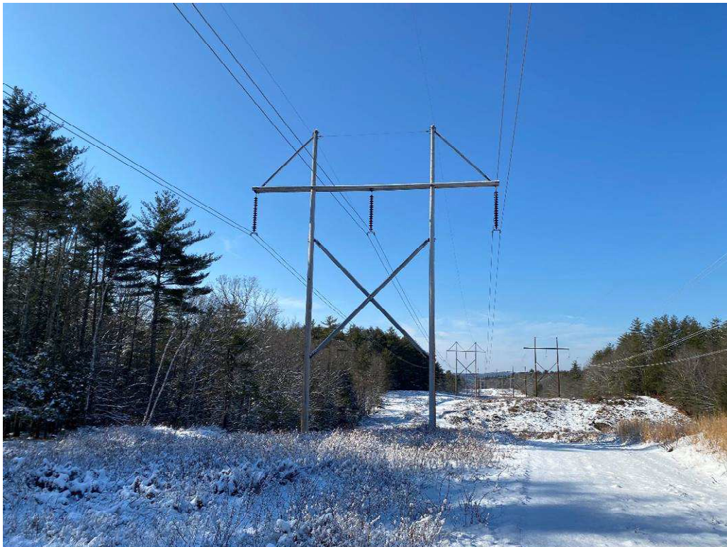
Photograph No. 58: Looking at proposed access and work pad location for 391 Structure 68.
