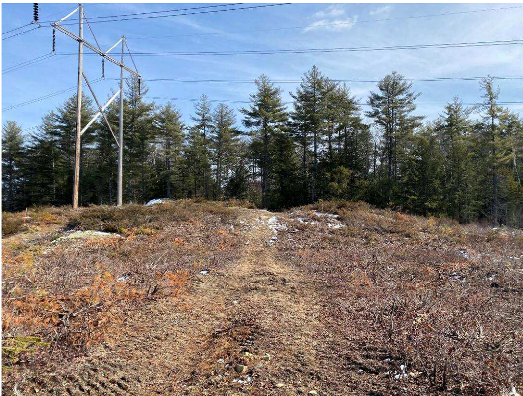
Photograph No. 22: Looking at proposed access and work pad location for 373 Structure 247.
