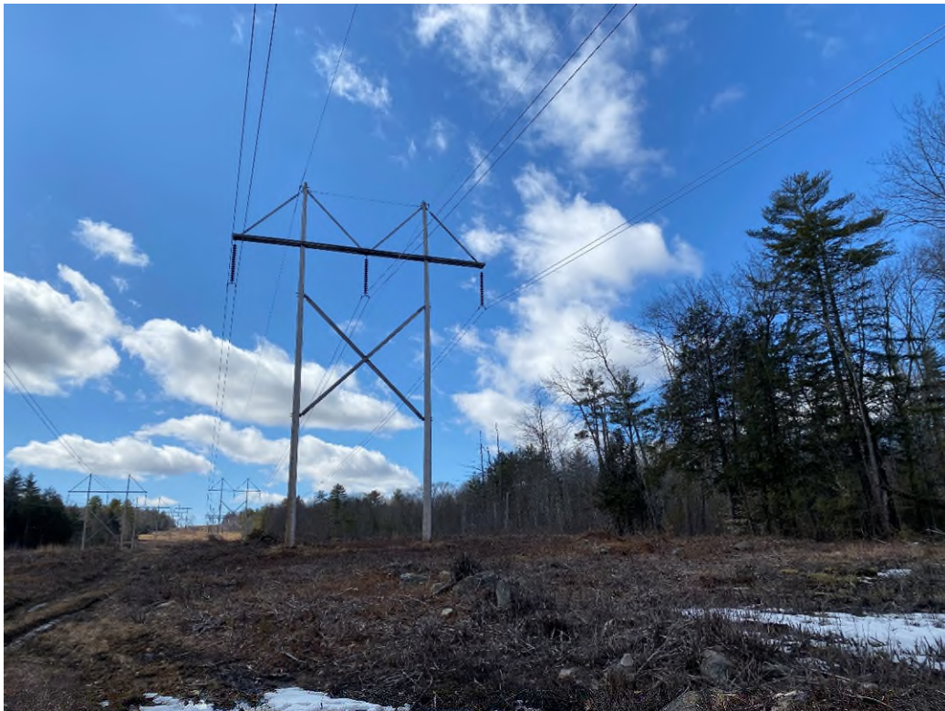
Photograph No. 64: Looking at proposed access and work pad location for 385 Structure 24.
