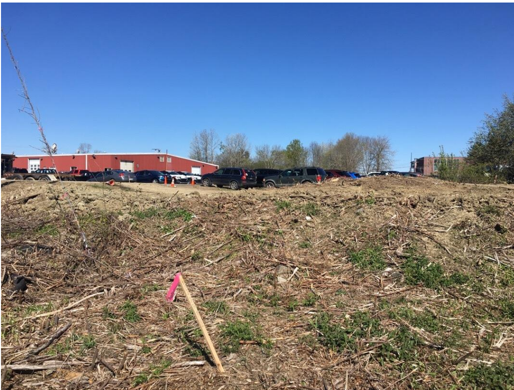
Photo 2. Future access point to F107 Str 137, view northwest.
