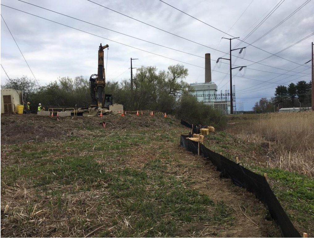
Photo 1. E194 Str 7- silt fence installation, view northeast.
