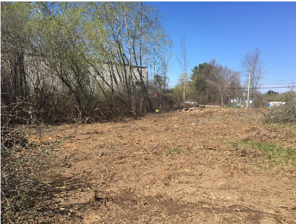
Photo 8. F107 Str 141- clearing for work pad, facing northwest.
