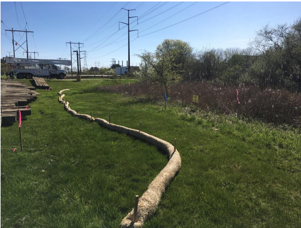
Photo 6. E194 Str 9/F107 Str 135- temporary straw wattle, view east.
