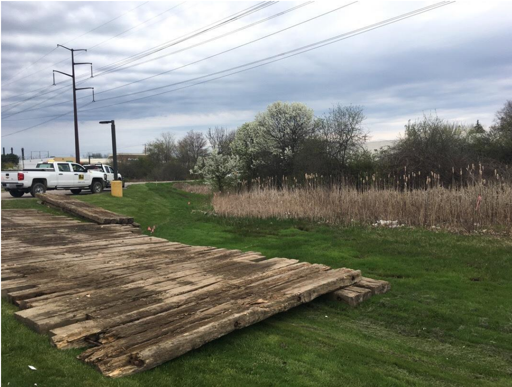
Photo 3. E194 Str 9/F107 Str 135- work pad, view southeast.
