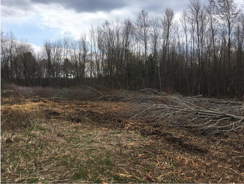
Photo 7. F107 Str 143- tree clearing for work pad, view south.
