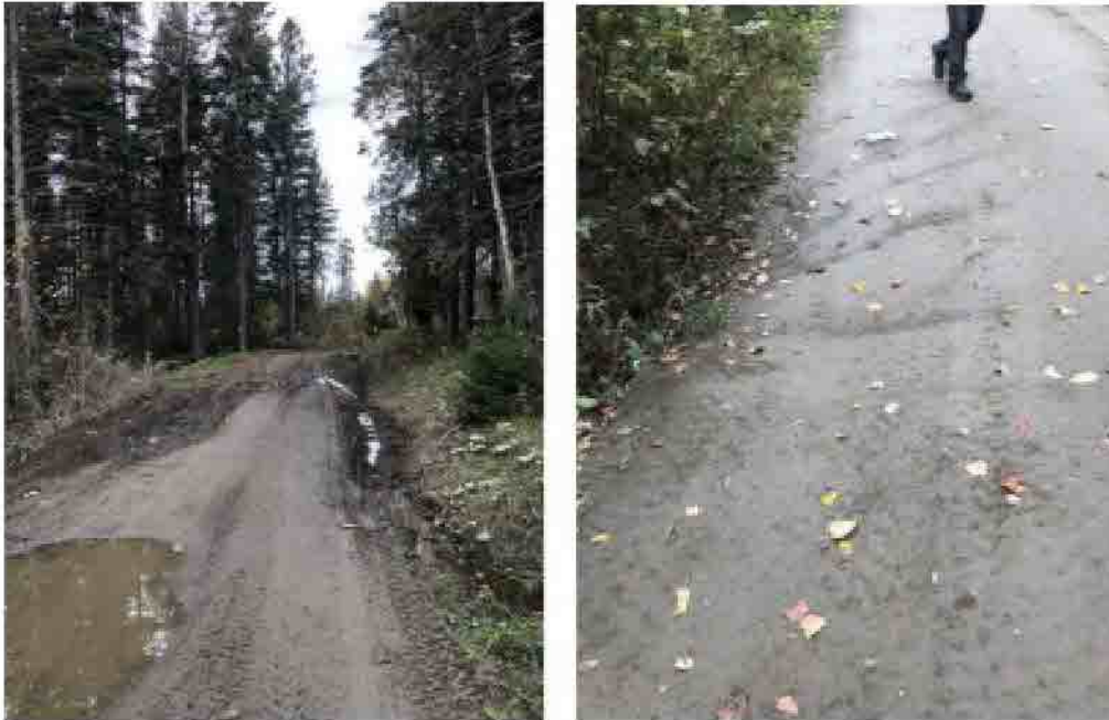
Figure 4- Mud on trail and ATV tracks in ditch and minor sedimentation on trail from water.
